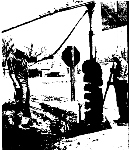
HOLES FOR TRAFFIC SIGNAL POLES were being dug Tuesday at 7th and Main Street by city street crewmen.
